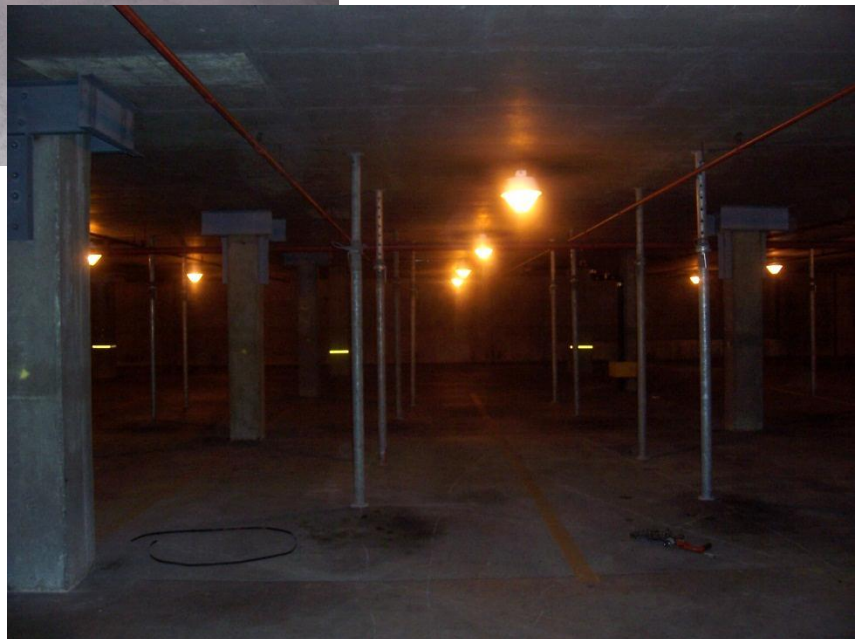
Temporary shoring and new shear head reinforcement at Commonwealth Garage
