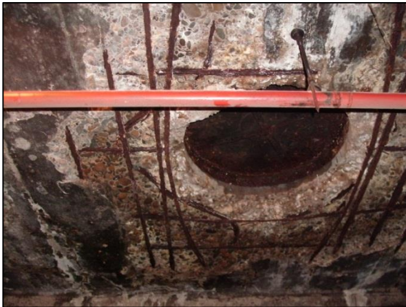
Deterioration of concrete slab and reinforcing due to age and heavy use of deicing salts on the drive surface above.
