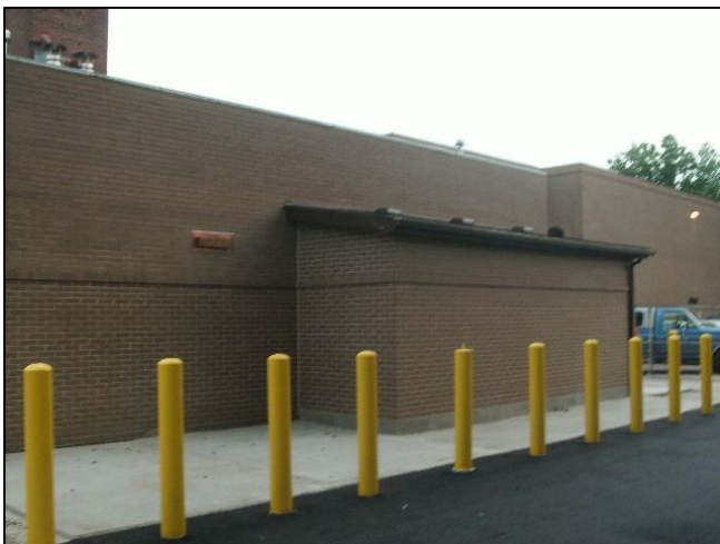
Reconstructed vault with new above ground access.
