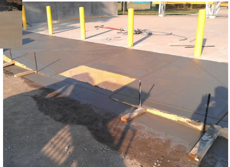
New sidewalk with ADA curb ramp.
