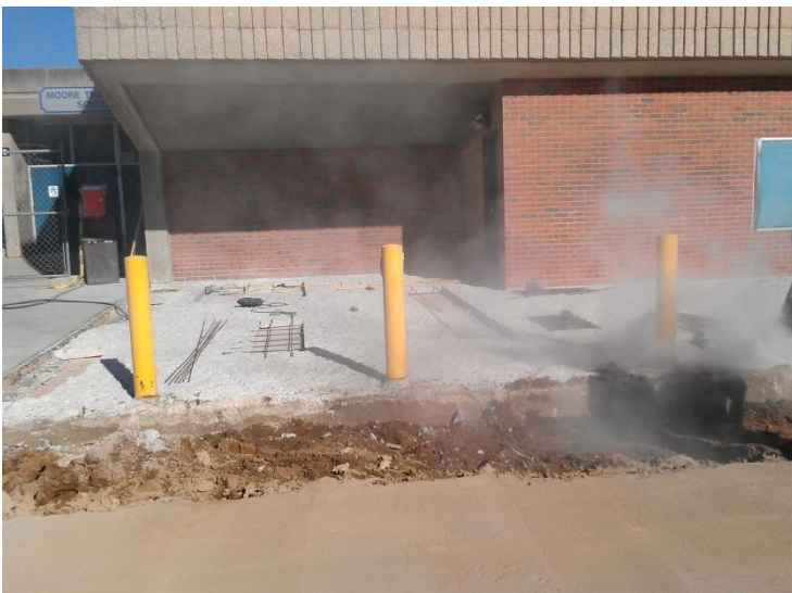
Demolition of deteriorated concrete at the tunnel slab top surface.
