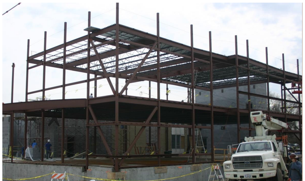
Addition under construction.
